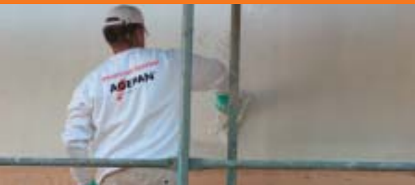
Direct plastering of the AGEPAN® THD T+G 230 at the facade.
